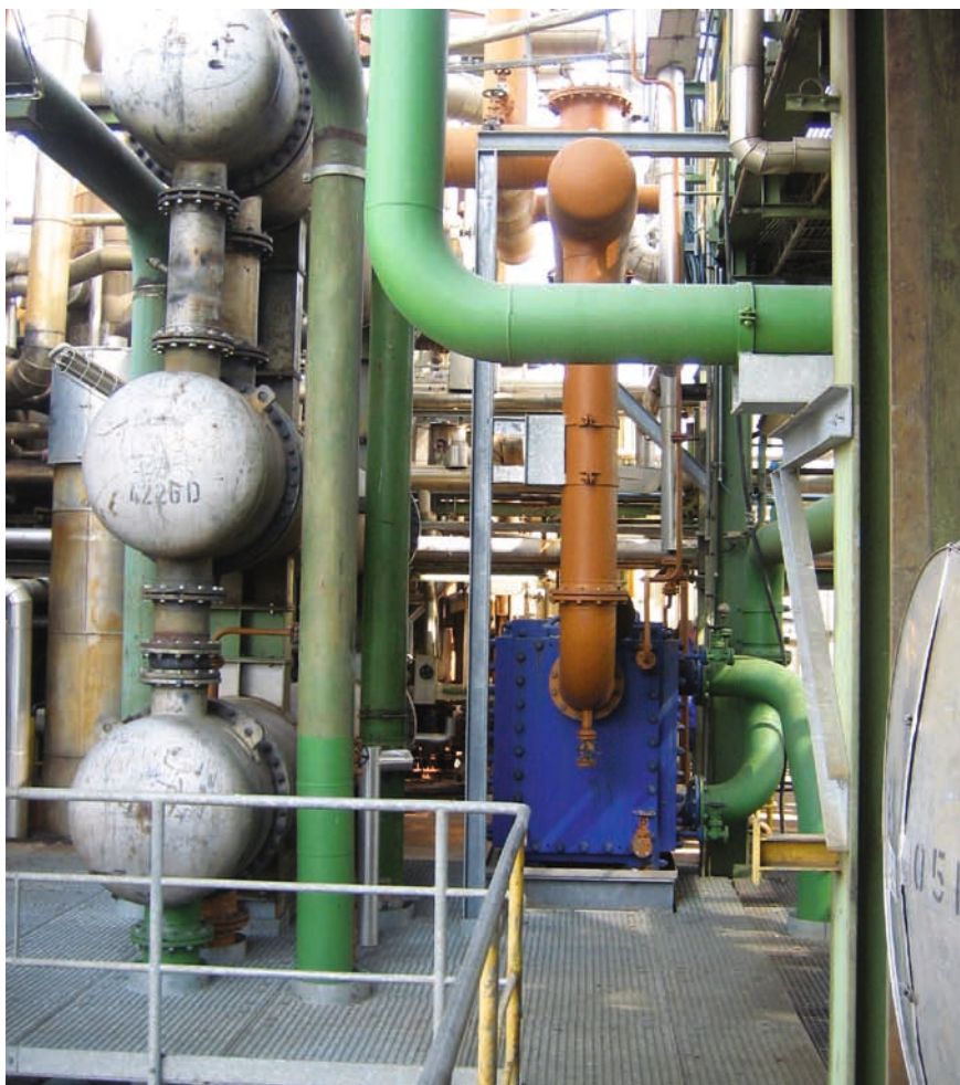
Figure 1. All-welded compact heat exchangers are very compact compared to shell-and-tube heat exchangers
