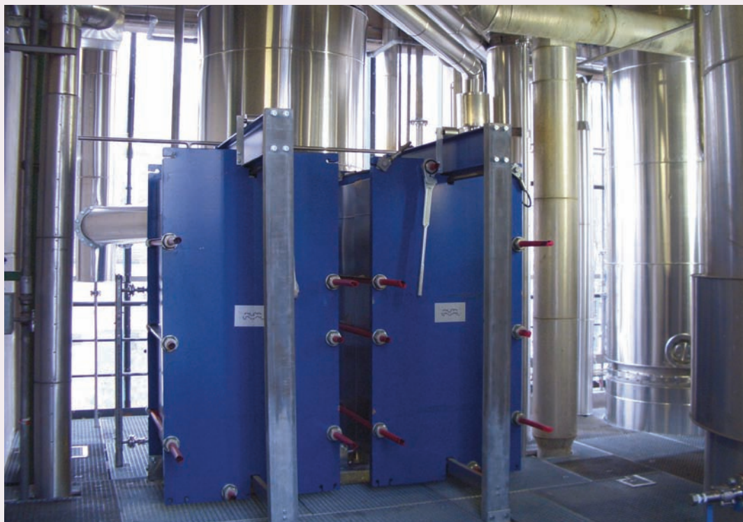
Compact installation of the reboilers on one floor
